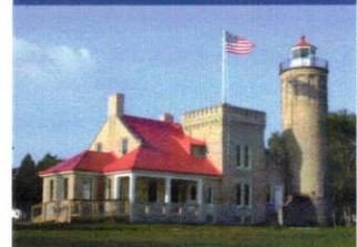
Mackinac Point Lighthouse
