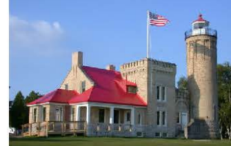
Mackinac Point Lighthouse
