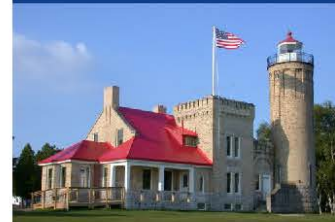
Mackinac Point Lighthouse
