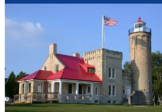
Mackinac Point Lighthouse
